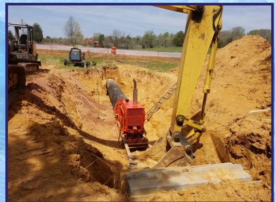
Boring I-85 for 24" water transmission line.
