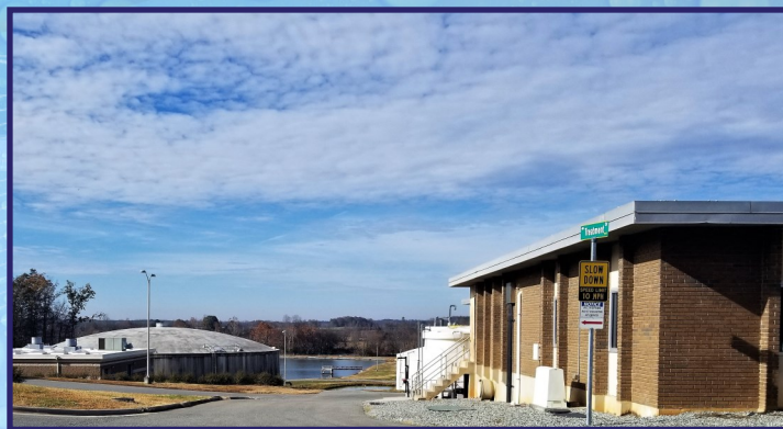
C.O. Pickle Plant (to the right) is currently being renovated.
