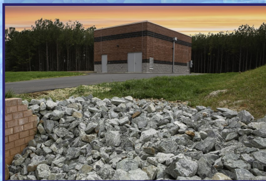
Hargrave Pump Station
