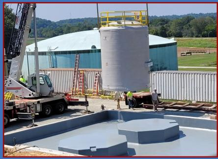
The image above shows one of two bulk tanks being placed by Omega Construction. Fiberglass reinforced plastic (FRP) tanks are less flexible and hold up well to bleach, making them a better choice for the chemical. The tanks are also resistant to UV light, giving them longer life. The tanks are anchored with bolts made of Hastelloy C, a product that stands up much better to corrosion than stainless steel. This project should be completed by the end of the year.
